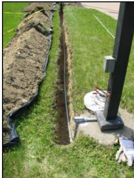
Another enlightening project was placing a light at the flag pole. It involved a trench to run electricity (see left), allowing illumination on the flag at night (See photo at right).
